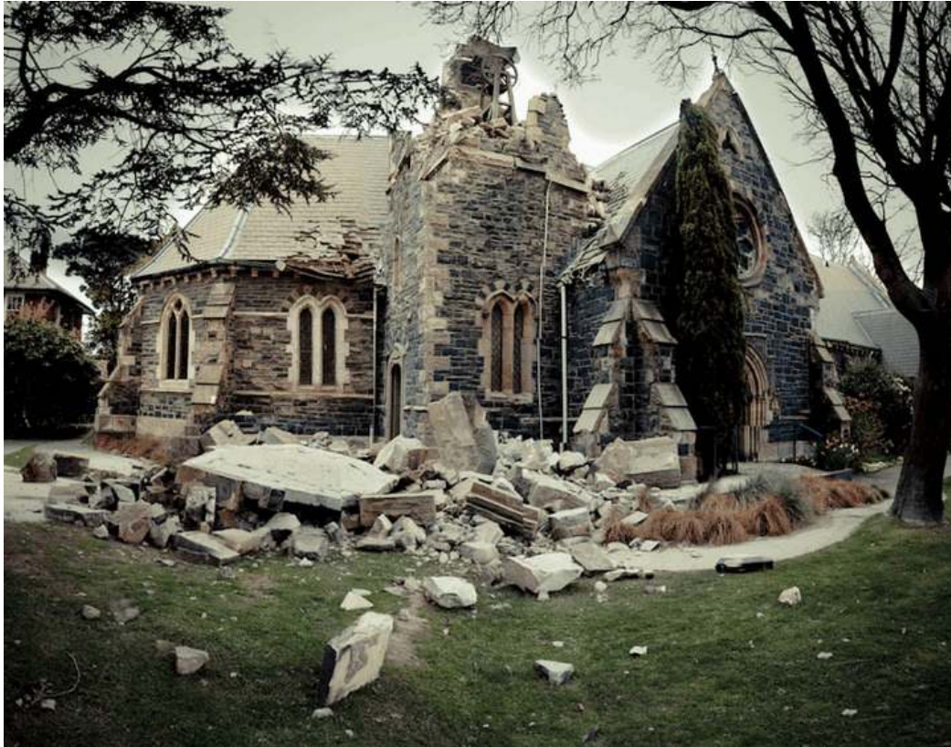
St. John's Anglican Church Bell Tower Destroyed
