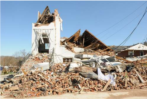
West Liberty UMC After Tornado
