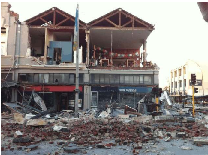
Facades Removed by Christchurch Earthquake
