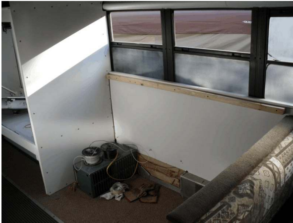
Space where Sink and Cabinet will Go
