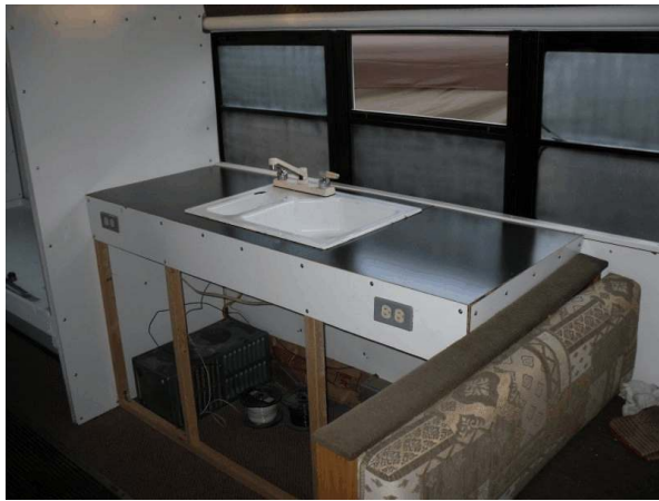
Sink in Place and Counter Top Added
