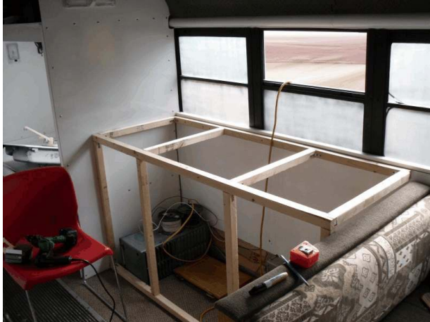
Sink Frame Built
