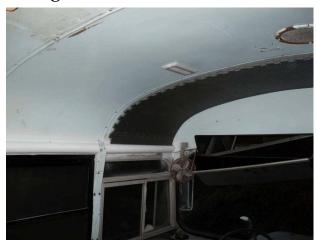
And here is the final piece in place for the first course of tile. I had to take a break from gluing tile at this point, for I needed to install a ceiling vent. I had salvaged a vent from the RV in Tennessee. There was previously a small round vent in the ceiling, which can be seen in these pictures, but it was inadequate, and had been painted completely shut up on the roof. I needed to cut a hole, and install the new vent, before putting more ceiling tiles up.
