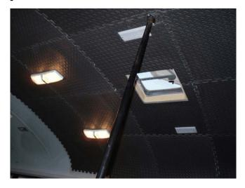
This photo was taken from the front step of the bus, looking in. It shows the vent installed, and several courses of tiles glued in place. You will also see four lights in place. Two are the original Carpenter Bus lights. They run off of the main battery. The others, which are lit, I installed. They run off of auxiliary power, or shore power and have switches on each light. These too were salvaged from the RV in Tennessee.
